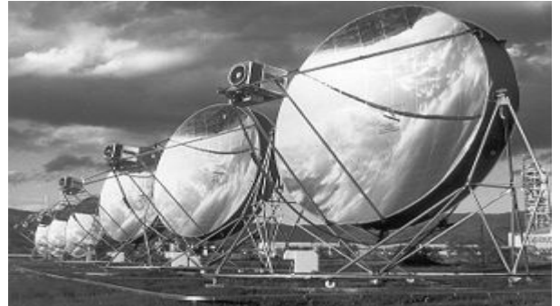
A parabolic dish and Stirling engine system, which concentrates solar energy to produce useful solar power.
